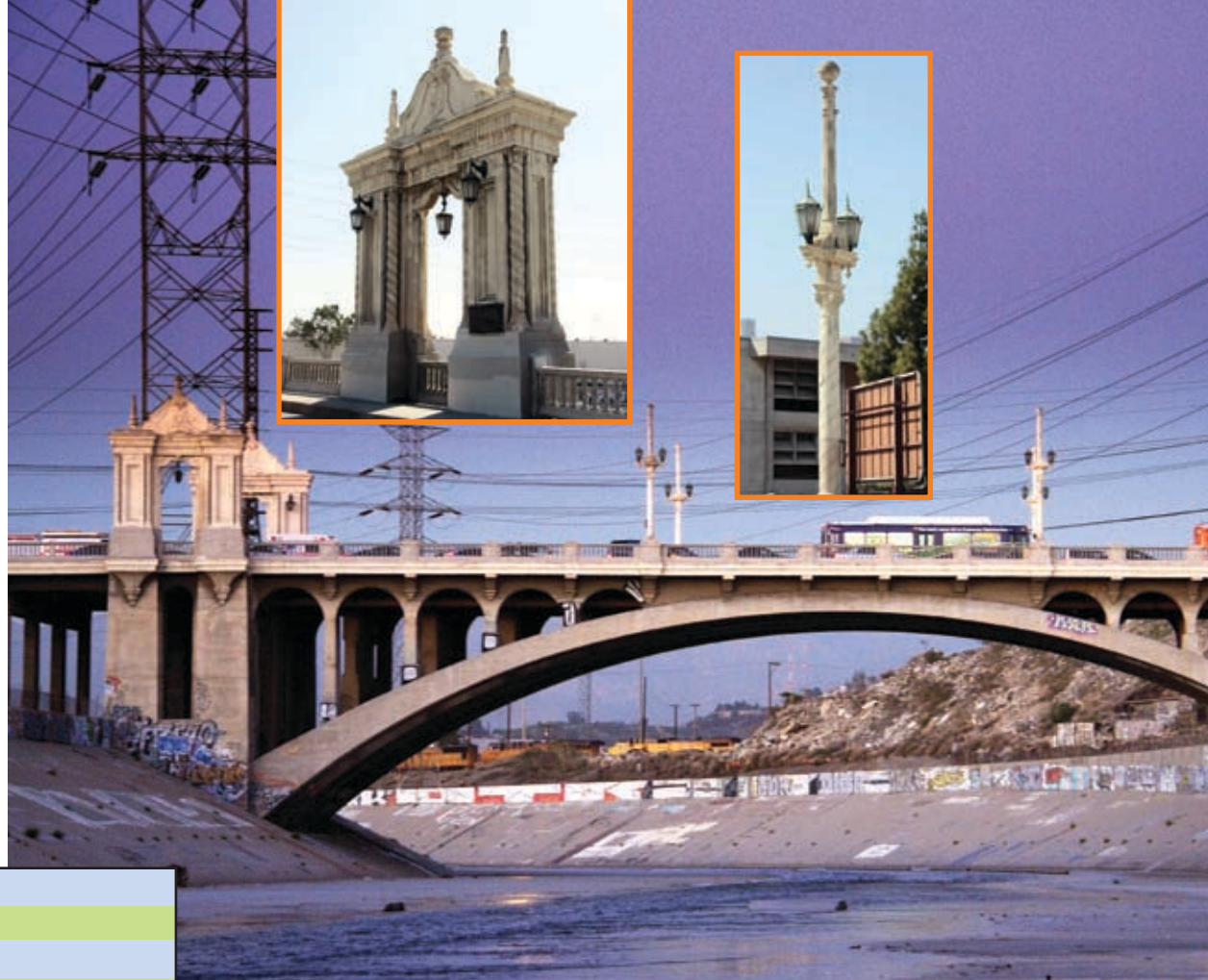
Opposite, top right: Former Macy Street Bridge, steel truss, c. 1926 (replaced)
