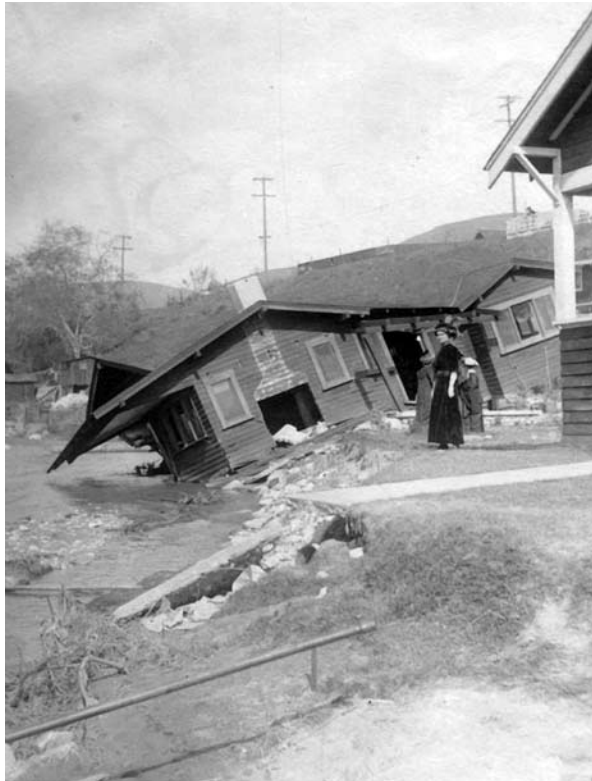
Homes along the Arroyo Seco in Highland Park overtaken by seasonal floods and erosion, 1913.
